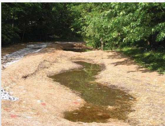
Biofiltration ponds protected with erosion mat facing west.
